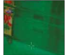
Thermal imaging showing the cold air staying inside the FX unit when the drawer is closed.
